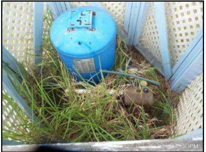
There is a well pump present in the backyard. It appears that the home was on a well at some point. This system does not appear to be in service at this time. Recommend further evaluation by a qualified contractor if buyer would like to use this for irrigation possibly.
