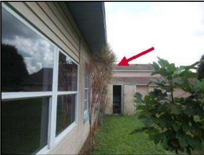
Prune or remove any plants that are in contact or proximity to home to eliminate pathways of wood destroying insects.
